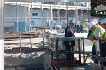
ECIS job site, Los Angeles, CA
